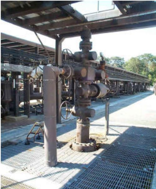
Oil and gas are extracted from beneath the Purbeck bedrock and Naturally Occurring Radioactive Material (NORM) accumulates where temperature or pressures change or where there is a disturbance to laminar flow. 'Tubulars', pumps, surface valves and vessels, are particularly susceptible to scale deposition. These require cleaning to reduce contamination to regulatory limits. Three problems exist:
